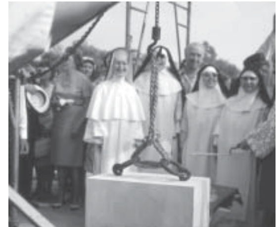
Adrian Dominican sister, Sr. Brigitta, joins our externs at the laying of the cornerstone in 1965
