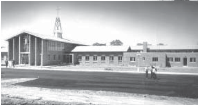
Facade during construction
