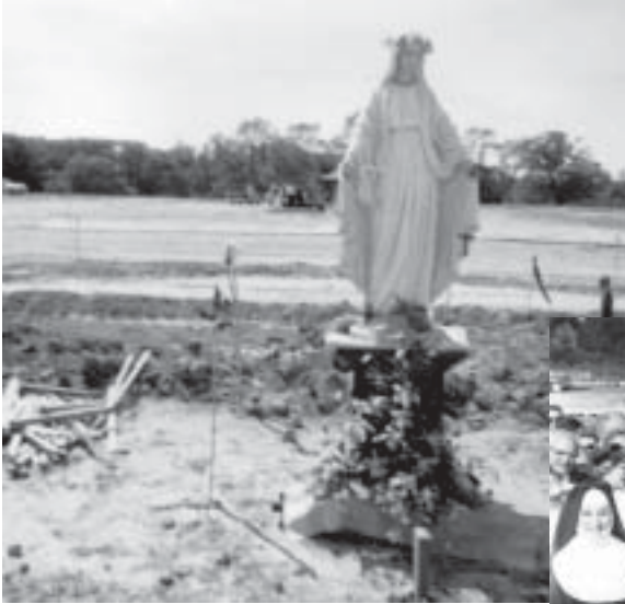
Our Blessed Mother oversees the construction
