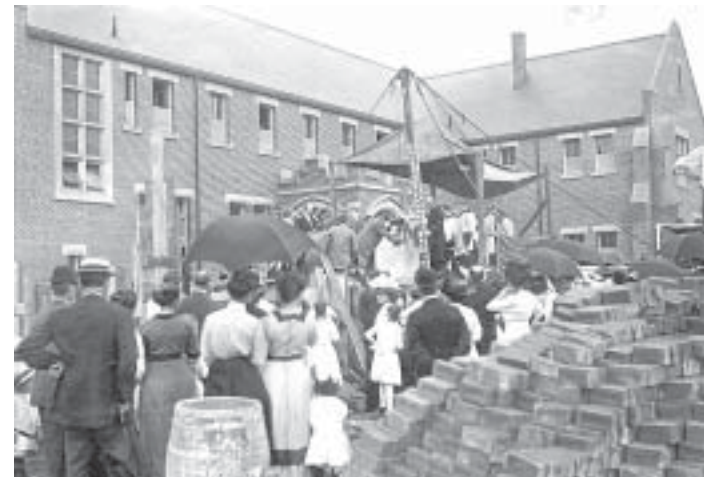
Laying the cornerstone
